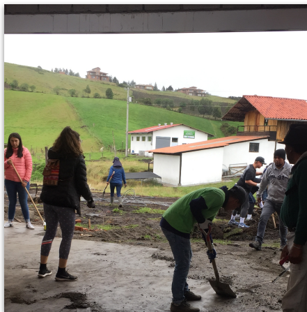
Scraping the concrete floors
