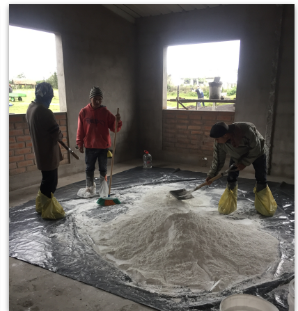
Mixing plaster for the walls
